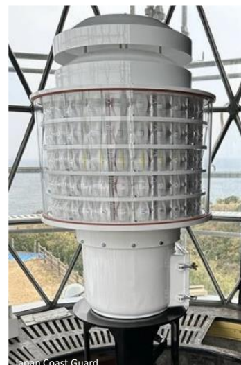
Newly installed LED Beacon
